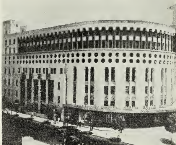
The Nippon Gekijo, one of the finest theatres in Tokyo, recently installed a Westrex advanced sound system, and was the first 3-D theatre there.
